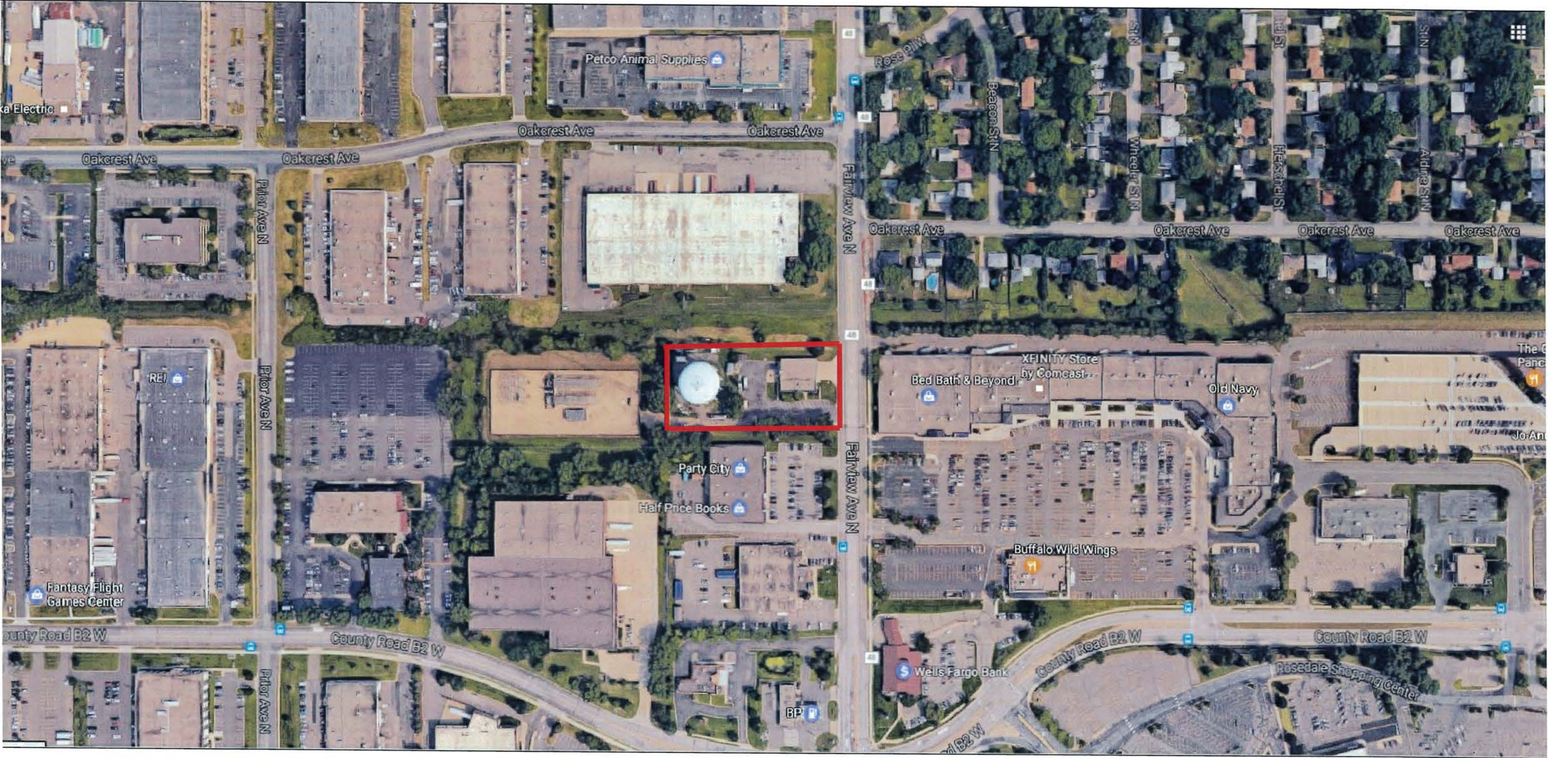
Aerial Roseville Water Tower Site
